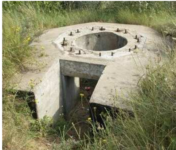
Fig. 2: Bunker without turret octagonal base plate. Screws for fixing the base plate are visible.
