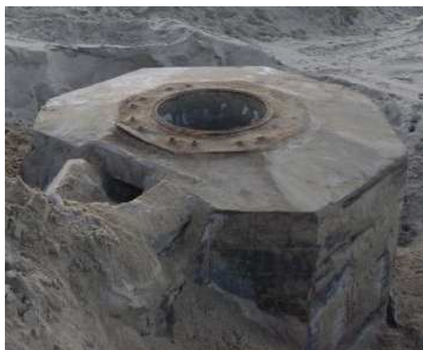
Fig. 3: Bunker with base plate and without turret
