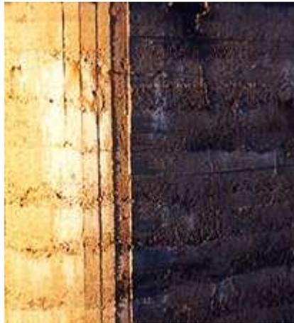
Fig. 1: wooden planks marks on the concrete structure
